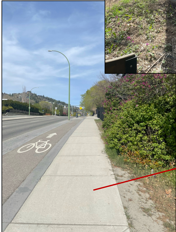
Sidewalk at Clifton Rd with completed ATC
