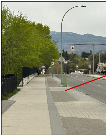
Sidewalk at Clifton Rd with completed ATC
