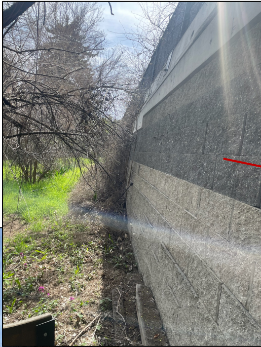
Retaining wall at Clifton sidewalk (from inside site)
